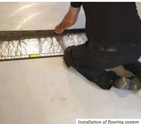
Installation of flooring system
